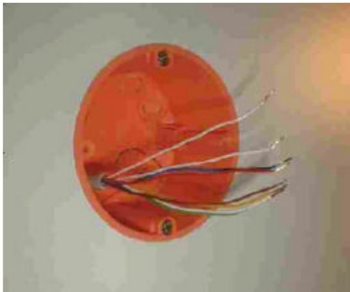
3. The sub-finery-socket (depth min. 40 mm) should be mounted smooth to the wall.
